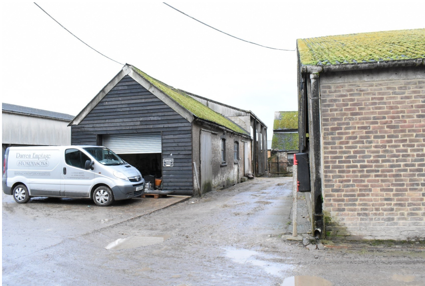
Plate 19: View of the original building in the south western range (facing NW)
