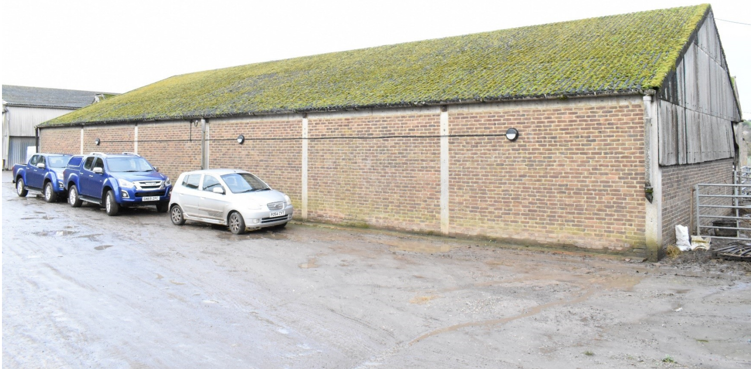
Plate 15: View of the rear building of one of the conversions (facing W)
