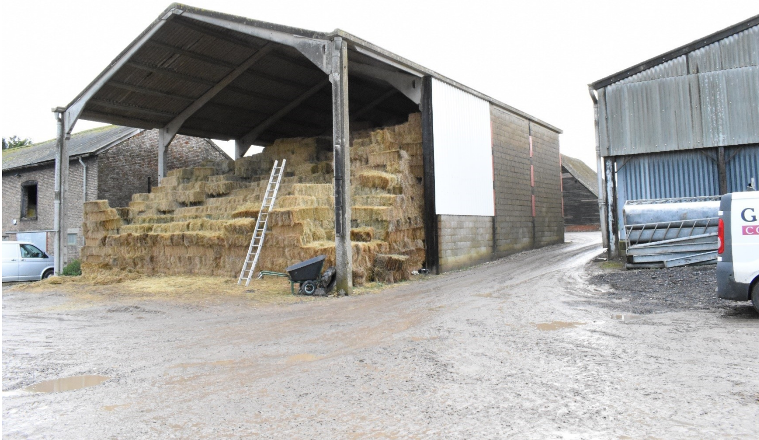
Plate 13: View towards the site of one of the proposed conversions (facing E)
