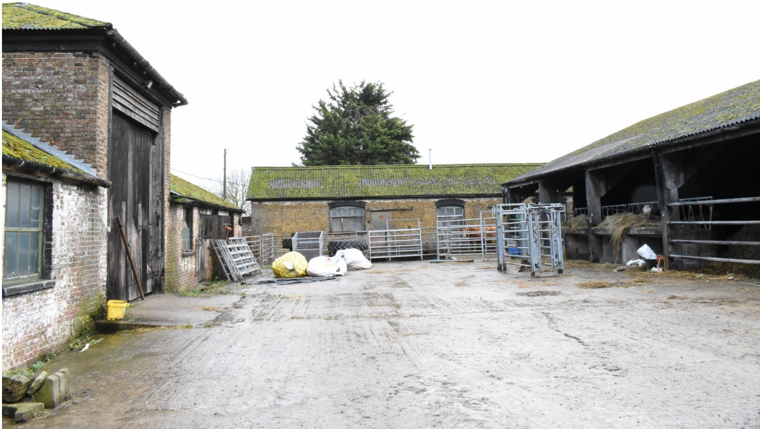
Plate 20: View across the yard (facing NE)
