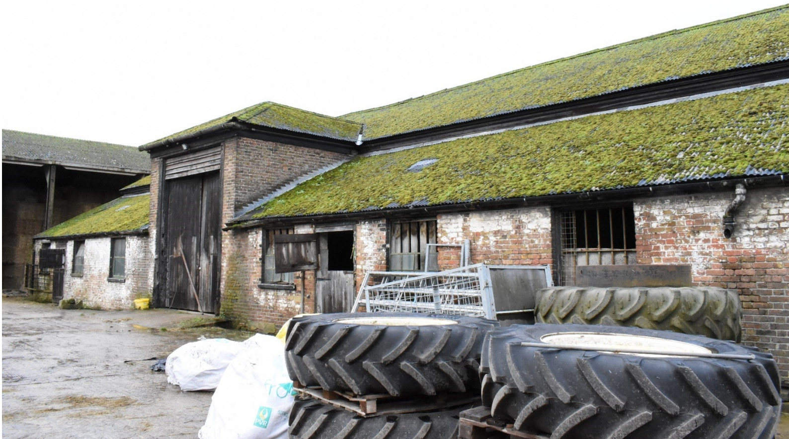
Plate 21: View of the barn on the north western range (facing W)
