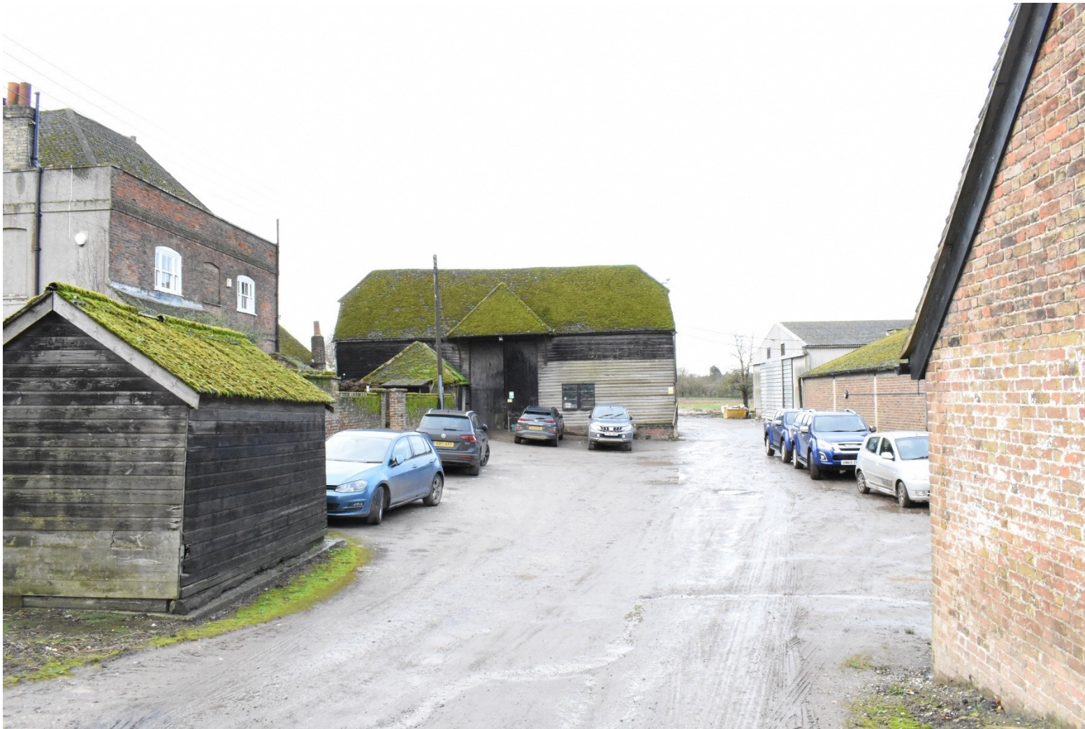
Plate 17: View across towards the Grade II listed house and barn (facing SW)
